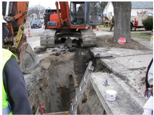
Picture to the left is Fife Avenue Project where 330 feet of 8-inch sanitary sewer was replaced.
